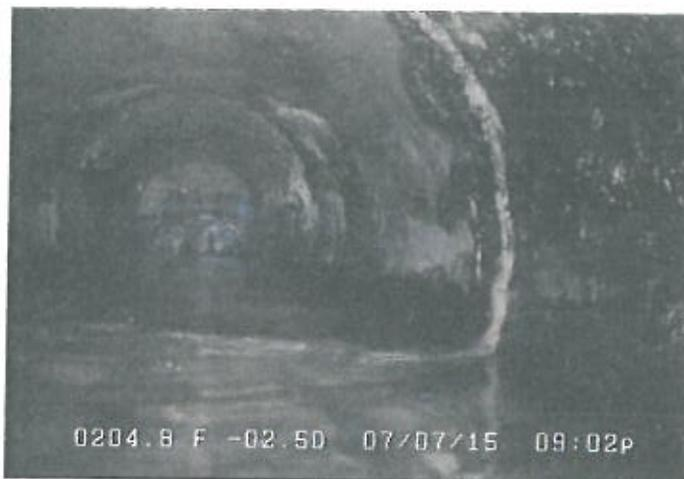
JS - Joint Separated @ 204.8 ft. WATER COMMING IN FROM JOINT
