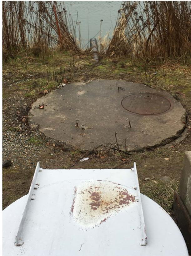
*Photo of Lift Station, wet well lid and overflow discharging pipe adjacent to the Clark Fork River.*
