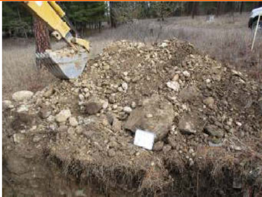
Test Pit (TP-2)
